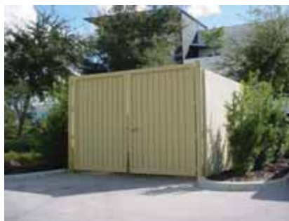
Enclosure constructed of stucco-finished concrete block with steel swing gates across full front of enclosure.
