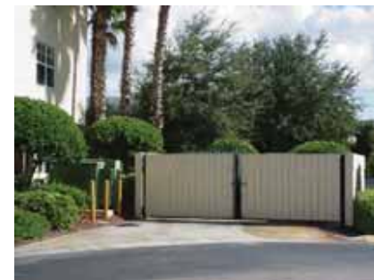
Dumpster enclosure constructed of stucco-finished concrete block with wooden-clad, steel frame swing gates.
